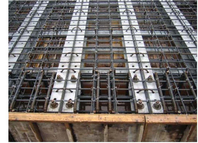
桁上面鉄筋配筋
