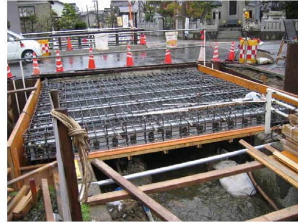
桁上面鉄筋配筋
